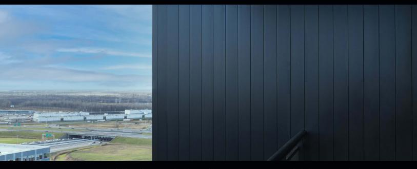
SH-09 is a plank-like siding entirely designed out of ultra-strong extruded aluminum and, as its name suggests, is moulded out of a single piece of metal, without any folding, giving it a distinctive look and texture.
